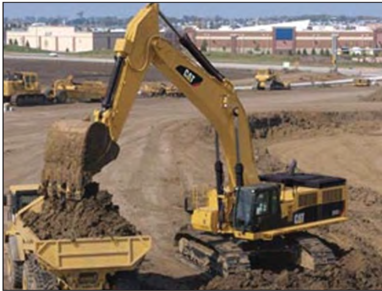
Figure 16-24: Excavator CAT 390D
